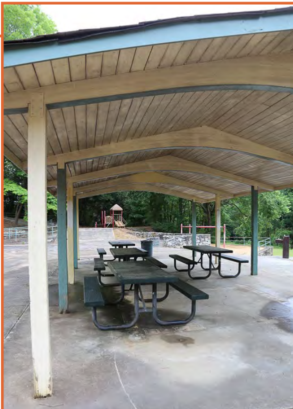
Top: remnants of a water features Below: pavilion and picnic tables Facing page: views of the upper and lower courts
